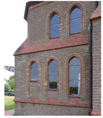
Closure of the building envelope by the protective glazing - the art glazing is simply placed in front from the inside after restoration.
