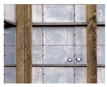
Fig. 2 - Glass sensor on the outside
