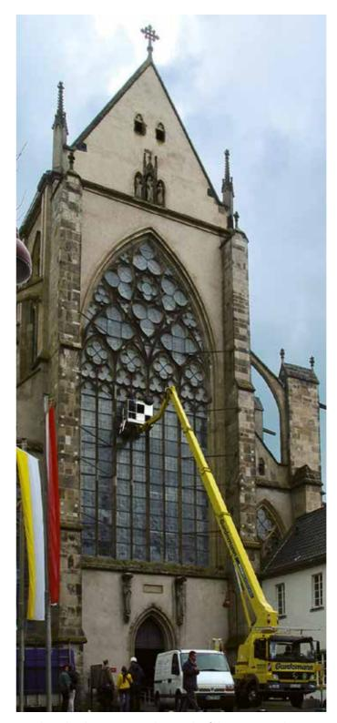
Attaching the glass sensors to the outside of the protective glazing
