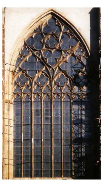
Installation of protective glazing with slightly frosted panels
